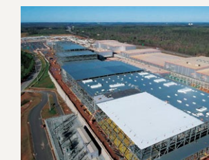
Construction site of the battery cell joint venture in North America
